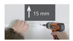
The top track must be mounted at least 15 mm from the ceiling with the curved edge downwards.
